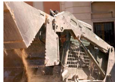
Spec. Espe Clothier, of the 821st Horizontal Engineer Company, West Virginia National Guard, 769th Engineer Battalion, 35th Engineer Brigade breaks ground at the Iraqi Police Training Facility in Furat, Baghdad.
